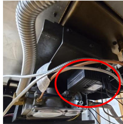
Figure 29 - Battery Installation
