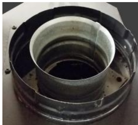
Vent Attachment Inspection – unbent and attached rings
