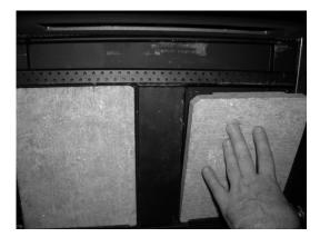
3) Place the left and right stones into the stove, exactly as shown-with the cut portion up and facing into the firebox.
