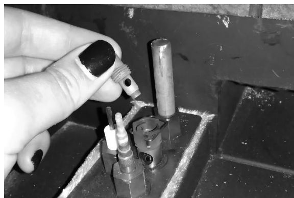
Figure 8 – Replacing Pilot Orifice
