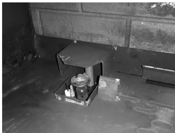
Figure 10 – Pilot, Shield, and Burner Position
