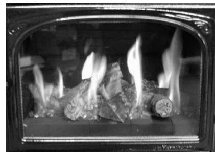
Figure 12 – Typical Flame Appearance
