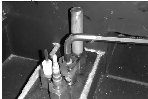
Figure 7 – Loosening Pilot Orifice
