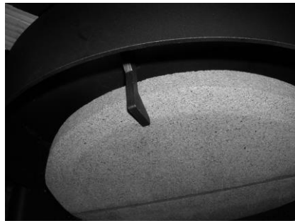
Figure 18 - Removing/Replacing the Baffle for Inspection
