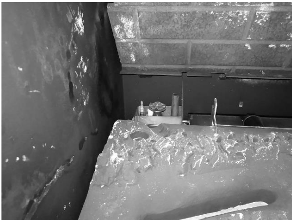
Figure 10 – Pilot, Shield, and Burner Position
