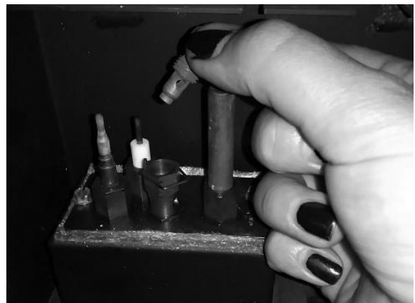
Figure 8 – Replacing Pilot Orifice
