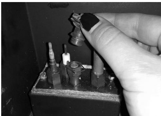
Figure 6 – Removing Pilot Burner Hood
