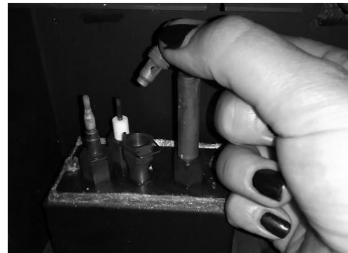
Figure 8 – Replacing Pilot Orifice
