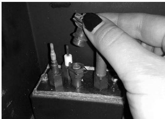
Figure 6 – Removing Pilot Burner Hood
