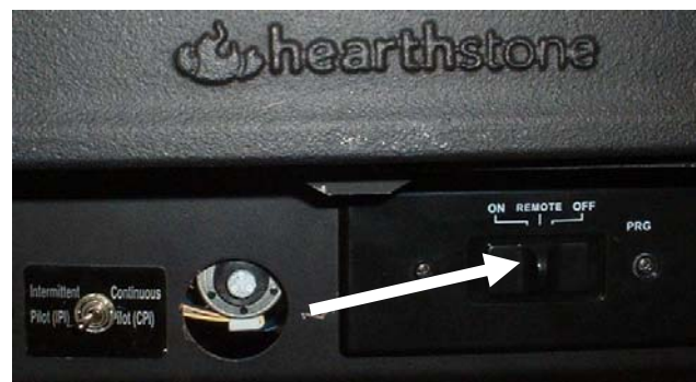
Photo 40 – DX Receiver Switch
