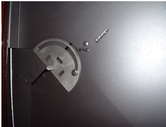
Photo 13: Restrictor Fully Closed
