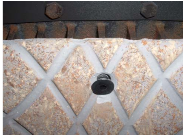
Photo 19 – Baffle Mounting Bolt
