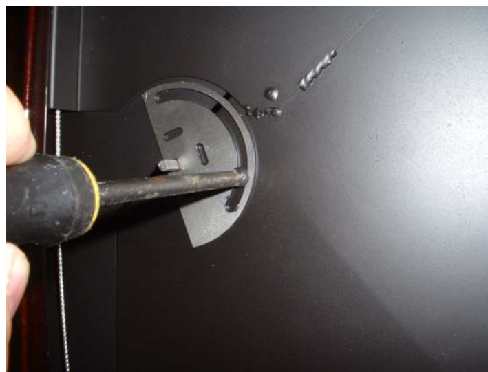
Photo 14: Restrictor Fully Opened (no restriction)
