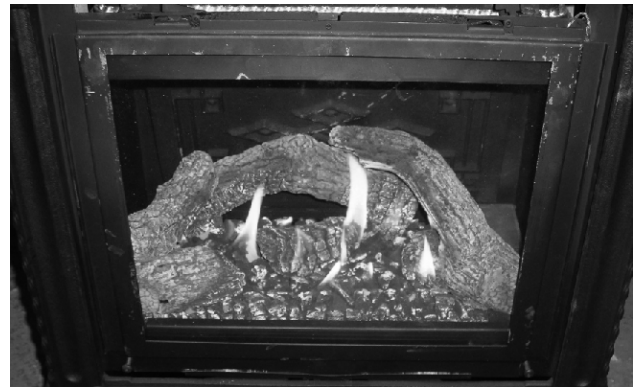
Figure 11: Typical flame appearance
