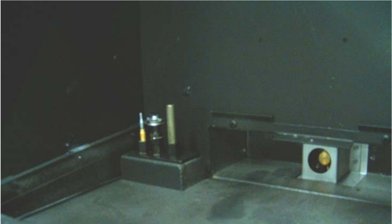
Photo shows Pilot assembly (left) and air shutter with burner orifice (right) in the firebox after the pan burner is removed.
