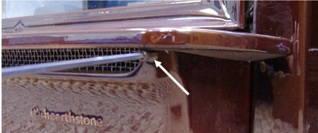
Photo #1: Removing the setscrew from the ash with the 5/32" allen wrench. One is located on the left and one on the right corner under the top edge of the lip.
