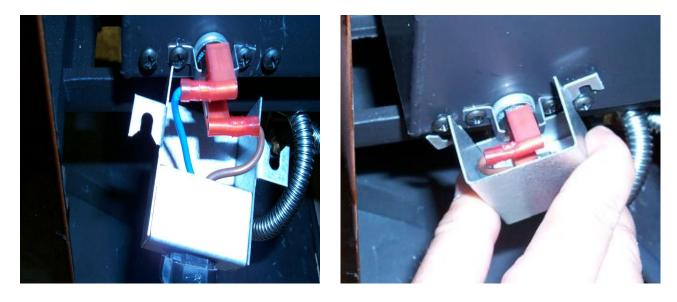
Photo #6 – Spade Terminal Connections
