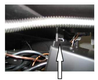
Photo #5 – Blower Tab Inserted in Mounting Slot
