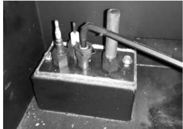
Figure 8 – Loosening Pilot Orifice
