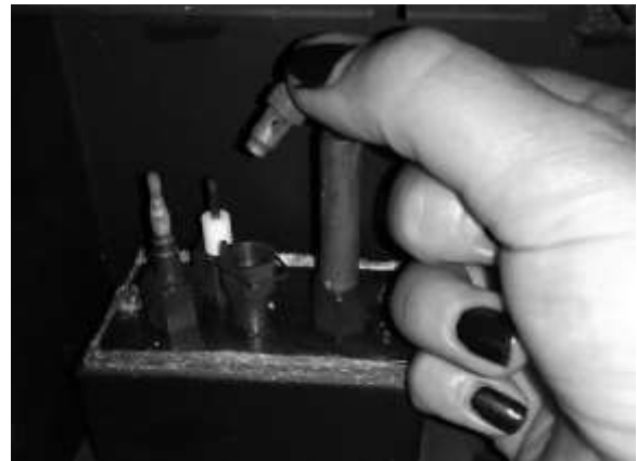
Figure 9 – Replacing Pilot Orifice
