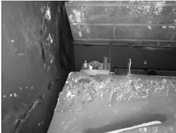
Figure 11 – Pilot, Shield, and Burner Position
