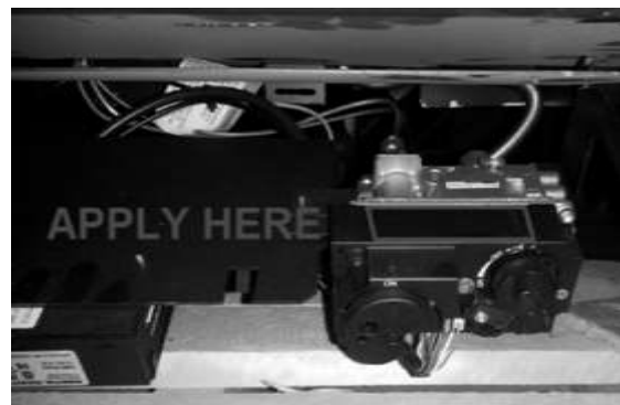
Figure 17 – Valve Warning Label Location
