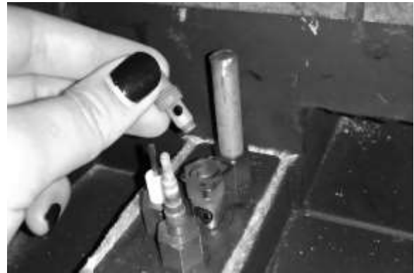
Figure 9 – Replacing Pilot Orifice
