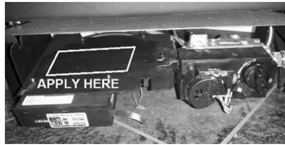
Figure 16 – Rating Plate Conversion Label Location
