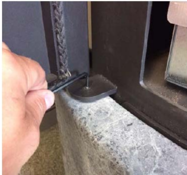
Photo #2: Turning in the setscrew on the top of the stone
