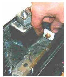
**Photo #11** - Place the white ceramic Gasket over the burner orifice.
