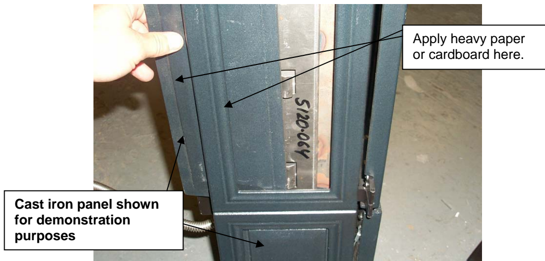
Figure 4 - Large Side Panel Installation
