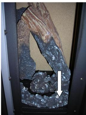
6. Slide the Right front ember strip next to the Left ember strip. The two fit together to hide the seam.
