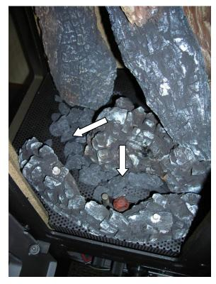
7. Sprinkle the charcoal embers over the burner ports. Ensure that you leave the ports open over the pilot, and where the main burner ignites.
