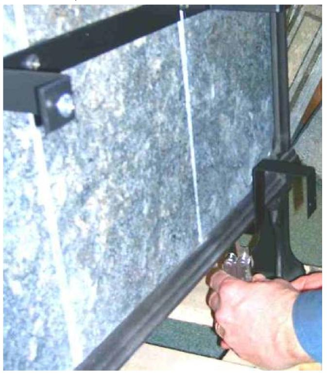
**Photo #3**Straighten the bottom clips and tighten the screws.
