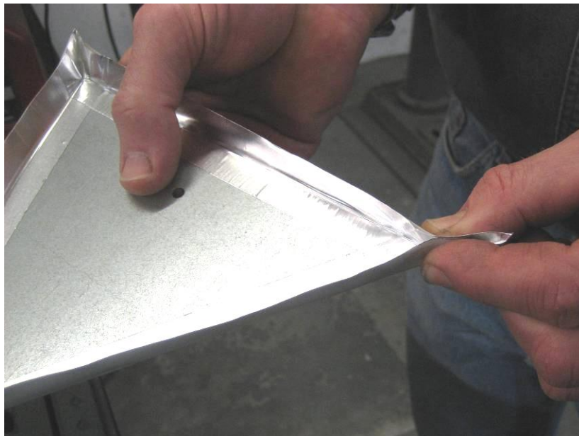
Figure 4 – 'V' crimping tape corners
