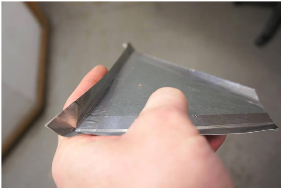
Figure 2 – Fold tape toward aluminum side
