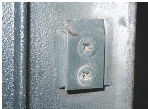
Figure 1 Latch keeper
