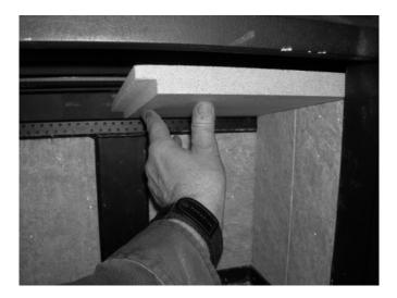
7) While lifting the rear portion of the right baffle, insert the left baffle by engaging the rear and tipping up the front. IMPORTANT – do not force the pieces as they could break or crack – they will fit together without forcing them into place. The two baffles will overlap at the center joint and sit in the grooves of the left and right stones.
