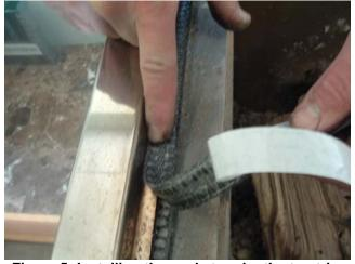
Figure 5: Installing the gasket under the top trim
