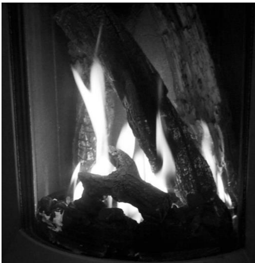
Figure 12: Typical flame appearance
