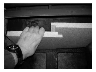
Figure 18 - Removing/Replacing the Baffle for Inspection
