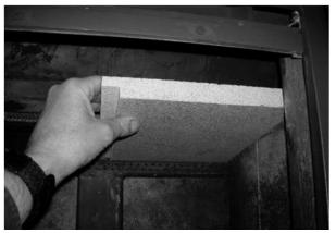
Figure 18 (cont.) - Removing/Replacing the Baffle for Inspection
